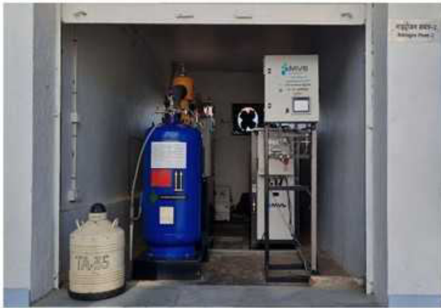
Figure 19 : The LN2 plant at Mount Abu Observatory, Gurushikhar, Rajasthan.
