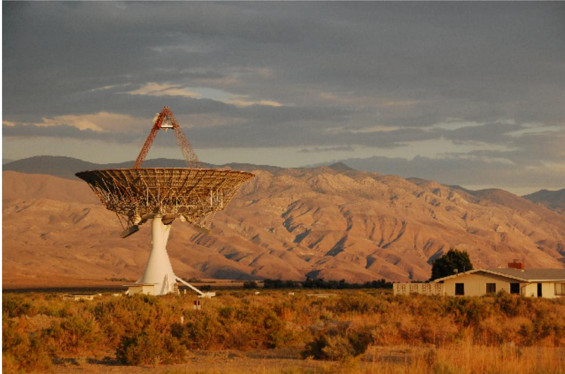
Figure 2.4: The Owens Valley Radio Telescope, 40 meter dish antenna, located near Big Pine, California, US. It is dedicated for blazar monitoring at 15 GHz.
