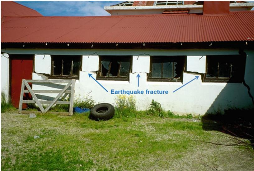
**Fig. 14.5** Earthquake fracture formed in the June 2000 earthquakes running through a building at a farm in South Iceland. The upper part of the building has moved to right relative to the lower part. This fracture is a strike-slip fault of type C. The same type of fault is seen in Figs. 8.3, 9.2, 13.7, 14.6 and 14.10
