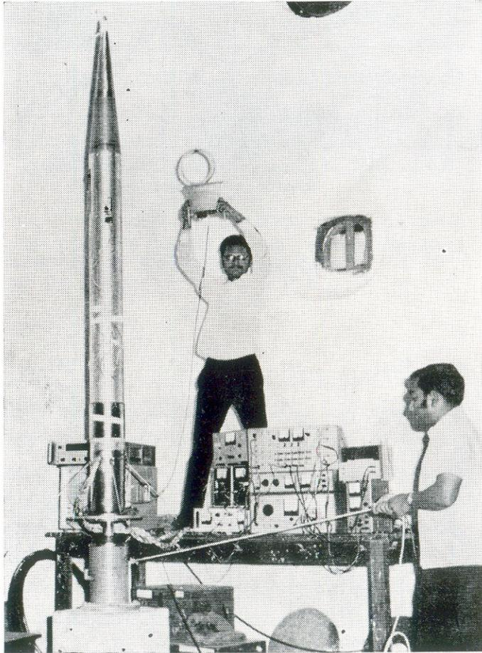
*Radio Propagation Receiver Payload calibration during shock test*
