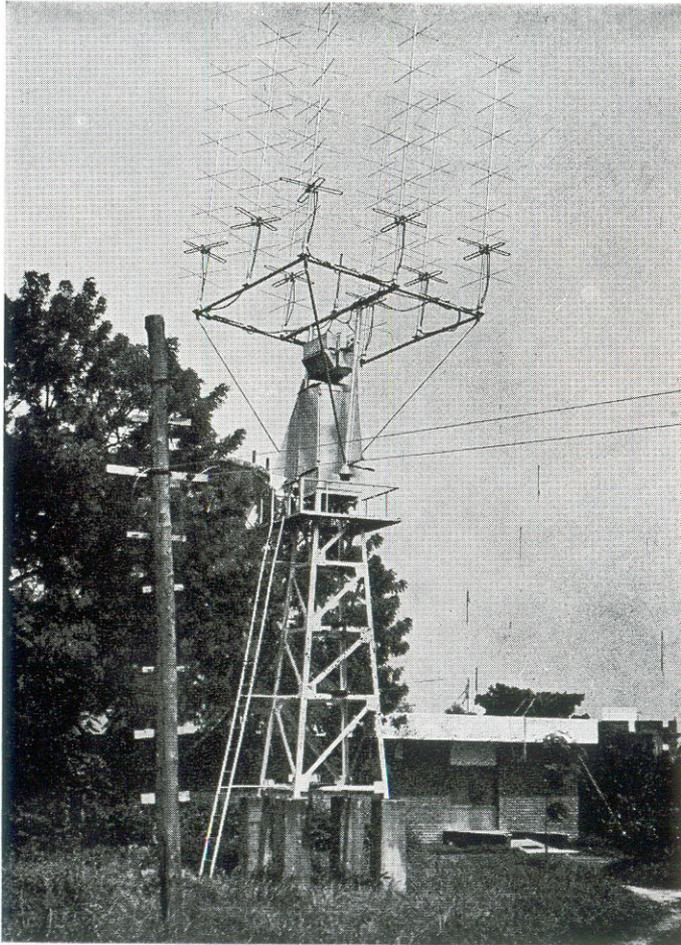
*Satellite Telemetry Antenna*
