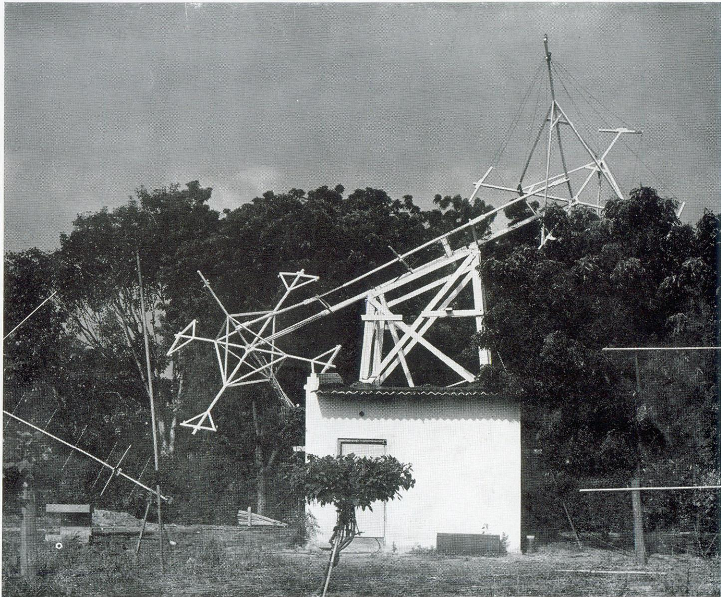
*Antenna for Solar Radio Spectrometer*
