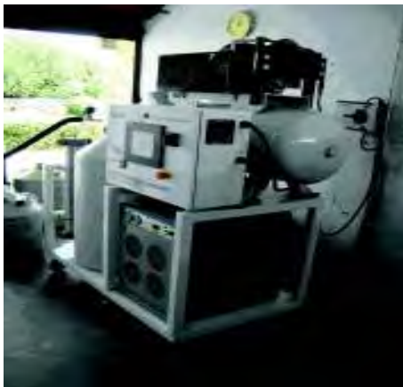
Figure 16: A small Liquid Nitrogen plant recently installed at Mt Abu Observatory at Gurushikar.
