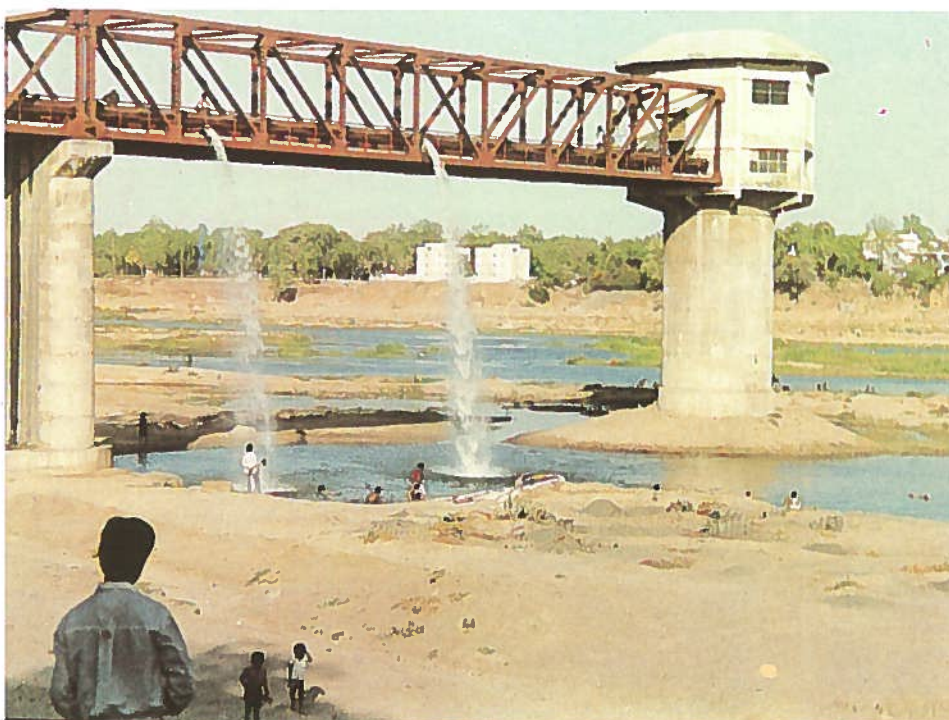
The bridge and the central collector well of the Sabarmati French well during tracer testing.
